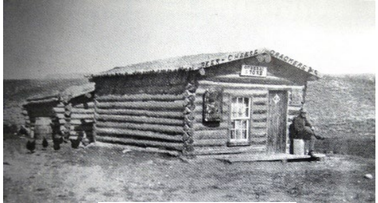
Selak Store and Post Office
