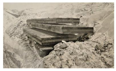
These mats were used to form a platform for the machine to operate on so that it might travel several feet above the ground on the snow and thus obtain clearance for the dumping of the bucket. The machine stood on three of the mats and as it passed on to the fourth and left the fifth, the crane picked up the fifth mat at the rear of the machine and placed it in front.
