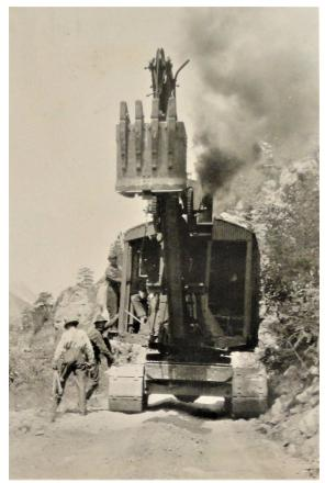
Two o'clock Sunday afternoon the large steam shovel of the National Park Service removed the last portion of the drift blocking the Fall River Pass. The shovel has been working almost continuously since May 15<sup>th</sup> and has handled an unusually large amount of snow.
