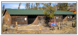
The roof of the Cottage Court was restored in October to prevent any further deterioration. Layers of existing roofing were removed, a few damaged one-inch boards were replaced with ones custom-milled at the Granby Sawmill, and slightly wider sheathing boards were added to form an overhang to protect the rafters from water damage. An ice and water shield was then covered with authentic 90 pound rolled roofing material. The Grand
